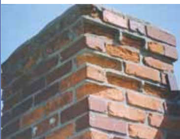
Severe spalling and deterioration is caused by water penetration.
